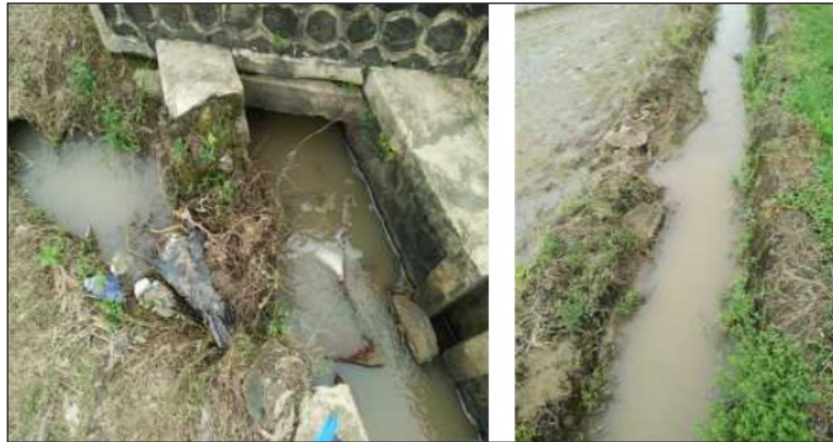
Figure 4. Channel conditions in the Punggur Utara irrigation area at Sumber Rejo Village
